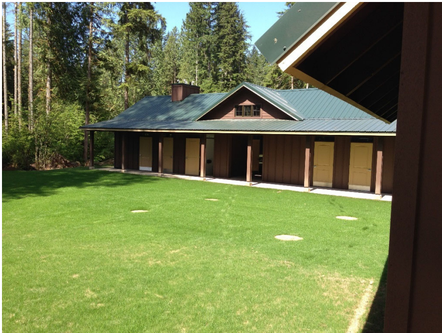
Restroom/Shower Building (individual shower/toilet rooms)
