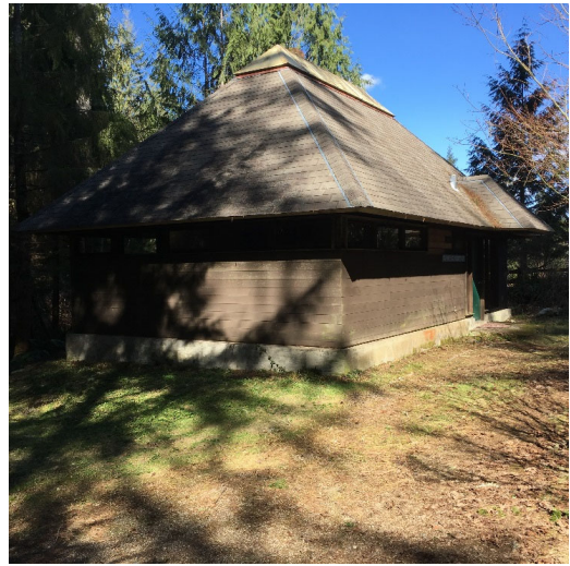
Staff Cabin (2 bedrooms-sleeps 4; bathroom/shower; kitchenette)
